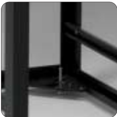
Welded corner post
