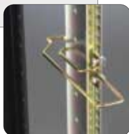
Cable hoop installed on rail
