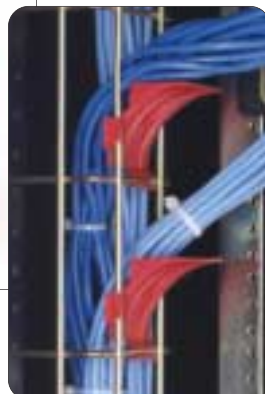
Installed cable drop outs
