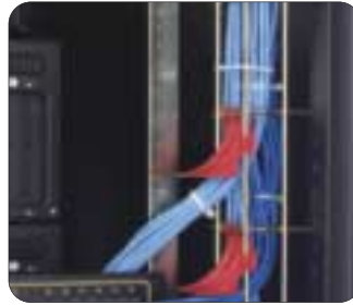
Installed vertical wire basket
